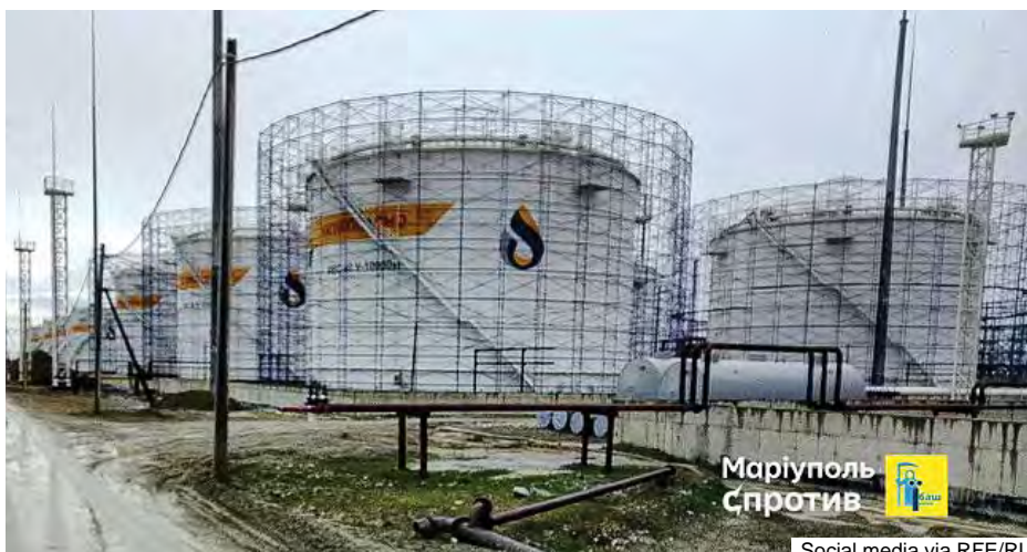
Oil tanks at the oil refinery in Slavyansk in Russia's Krasnodar region are seen with exterior metal cages meant to protect them from drone attacks.
