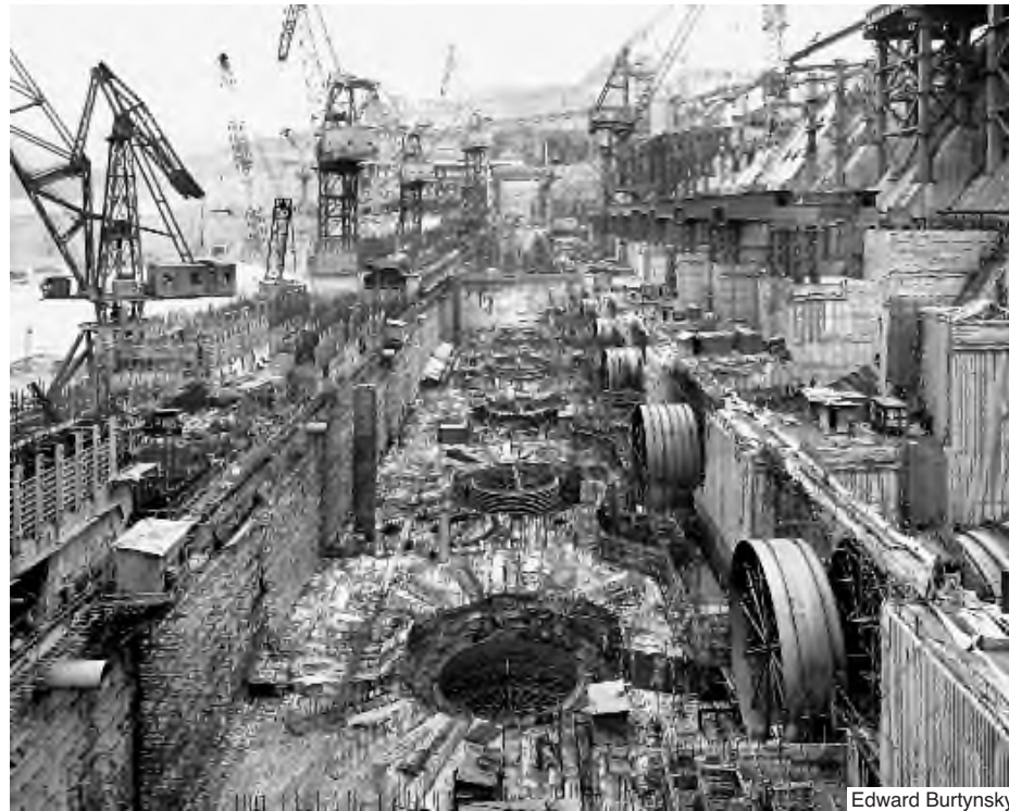
Three Gorges Dam Project, Yangtze River, China.
