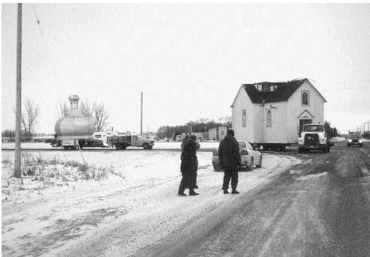
The building and dome of St. Nicholas Ukrainian Orthodox Church of Arbakka, Manitoba, are transported on flatbed trucks to Fort La Reine Museum in Portage La Prairie, some 200 miles away.
