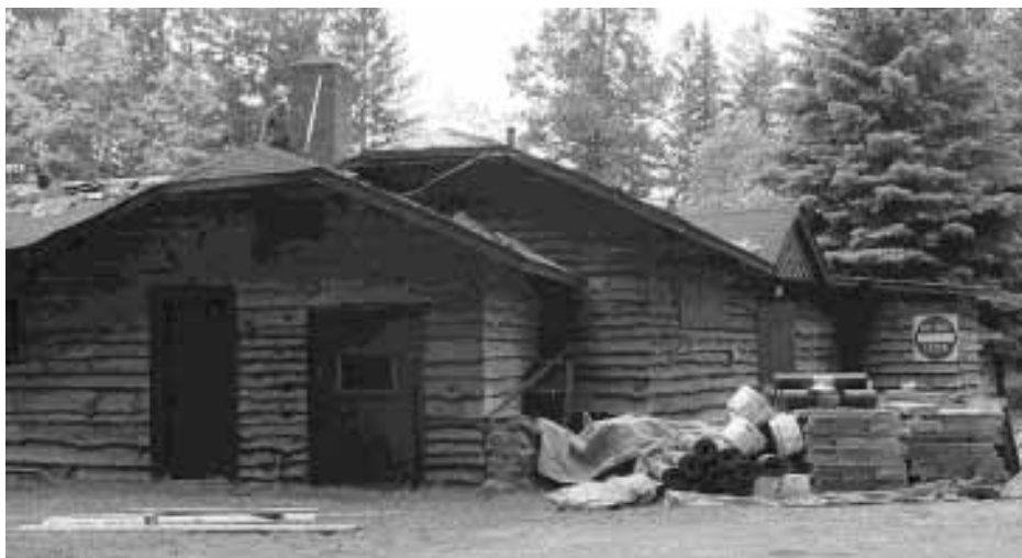
The studio, soon to be renovated inside, gets a new roof.
