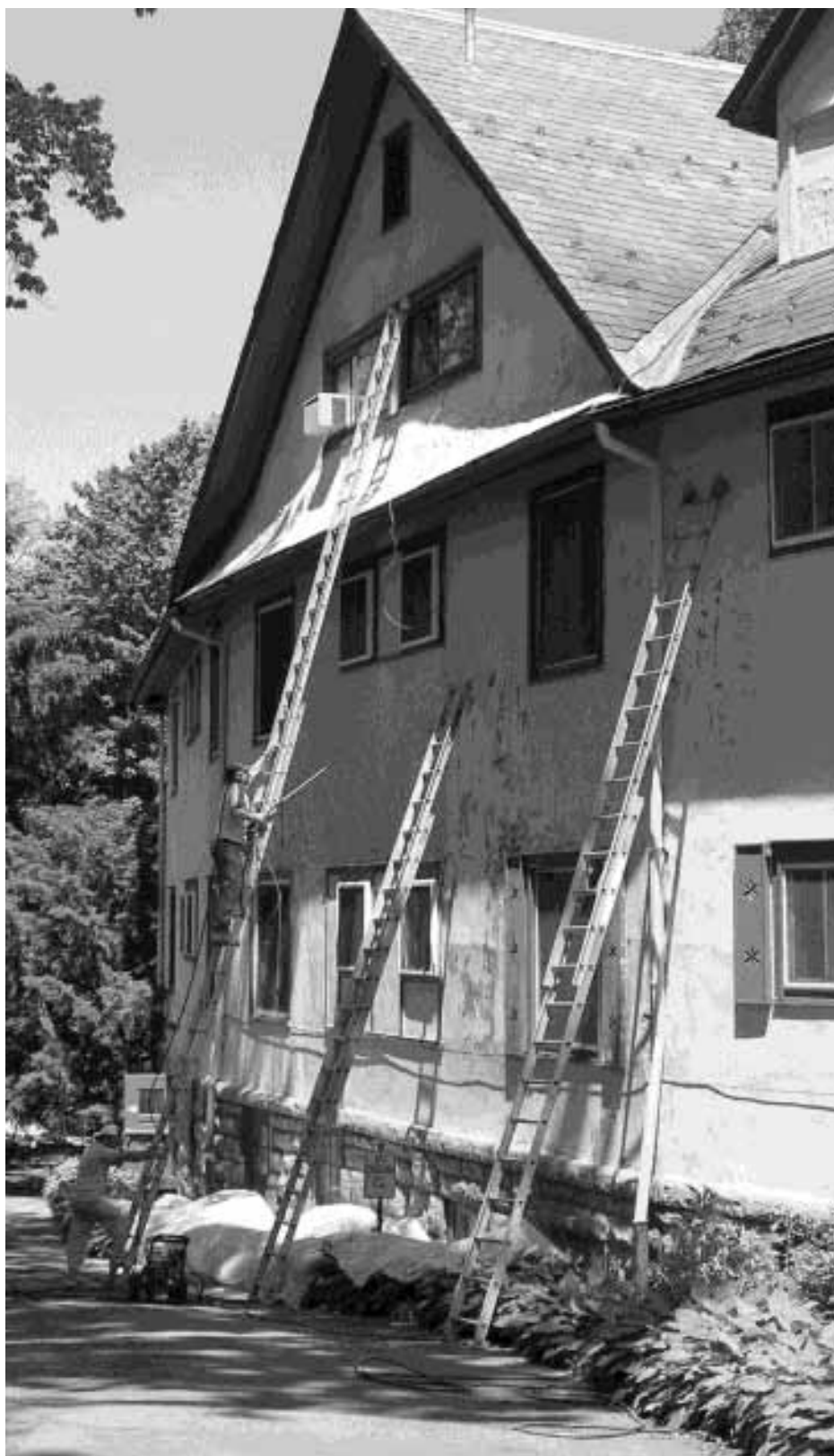
Soyuzivka's Main House gets prepped for a fresh coat of paint.
