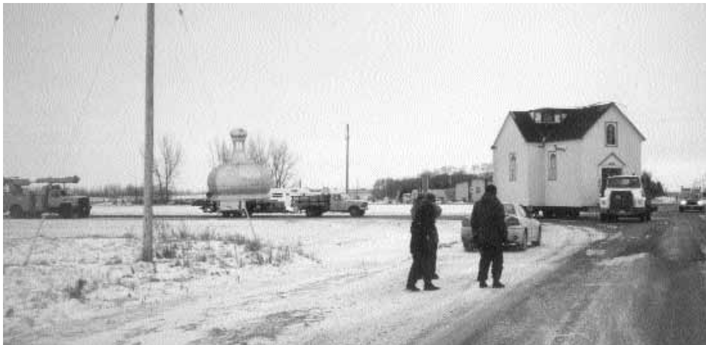
The church and its dome are moved, separately, on flatbed trucks to the Fort la Reine Museum grounds.
