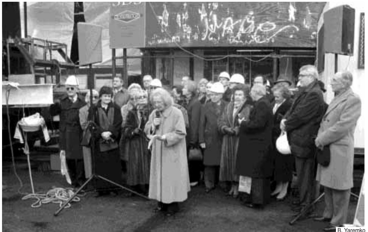
Board members, staff and friends of The Ukrainian Museum gathered at the construction site of the new building during the topping out ceremony on December 8. At the microphone is Olha Hnateyko, president of the museum's board of trustees.
