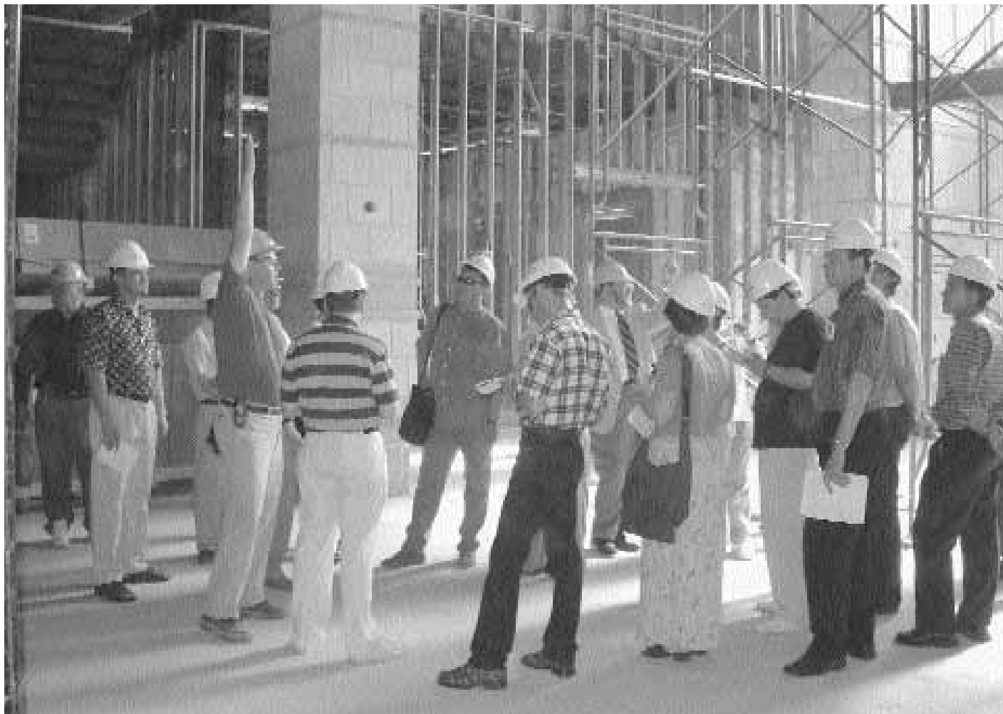
Neil Kluender of the Dugan & Meyers construction company directs the Kharkiv group’s attention overhead as he explains methods being used in the new municipal center under construction in Mason, Ohio, outside Cincinnati.
