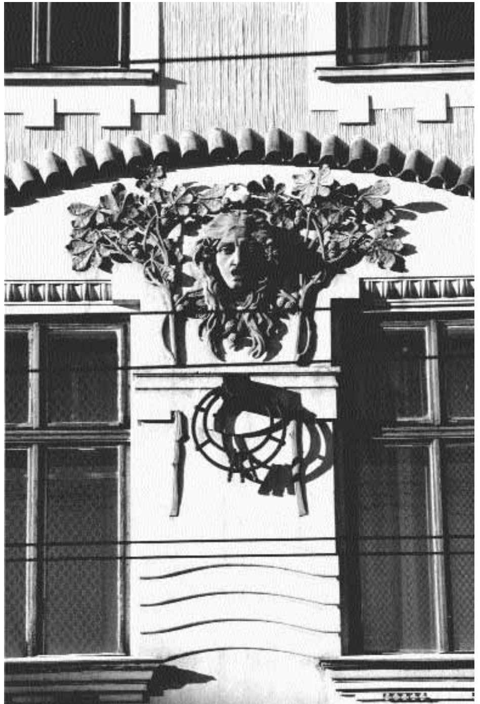
Mask and metalwork at a tenement house, 8 Rustaveli St., by Edmund Zuchiwiicz Co., 1905-1906.
