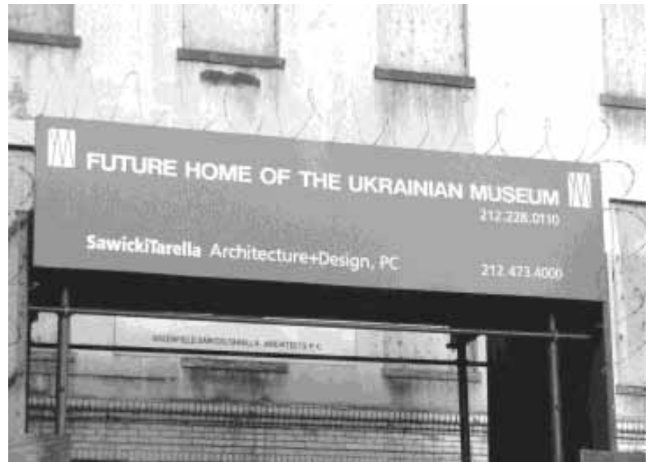
Scaffolding in front of existing structure heralds the beginning of construction of the new home for The Ukrainian Museum.
