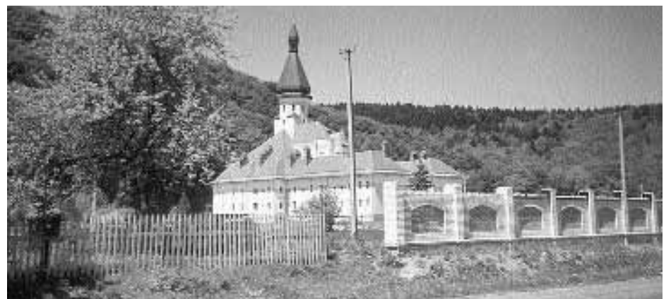
A view of the sisters' monastery under construction in Hoshiv.
