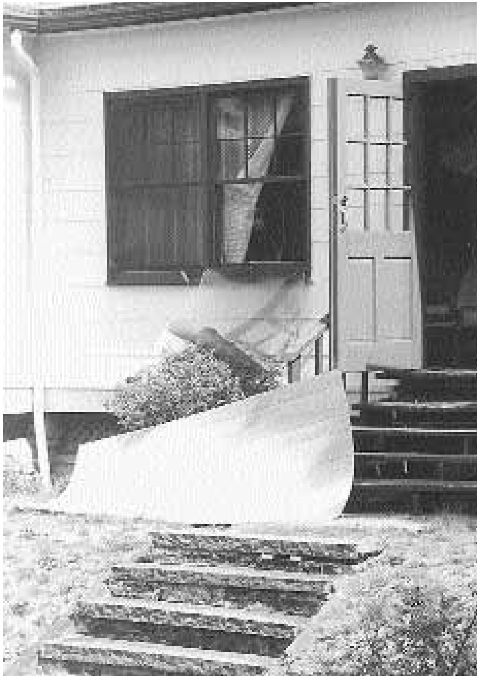
Destroyed particle board, a torn out screen and a broken window by the side entrance of the main building at the Verkhovyna resort.
