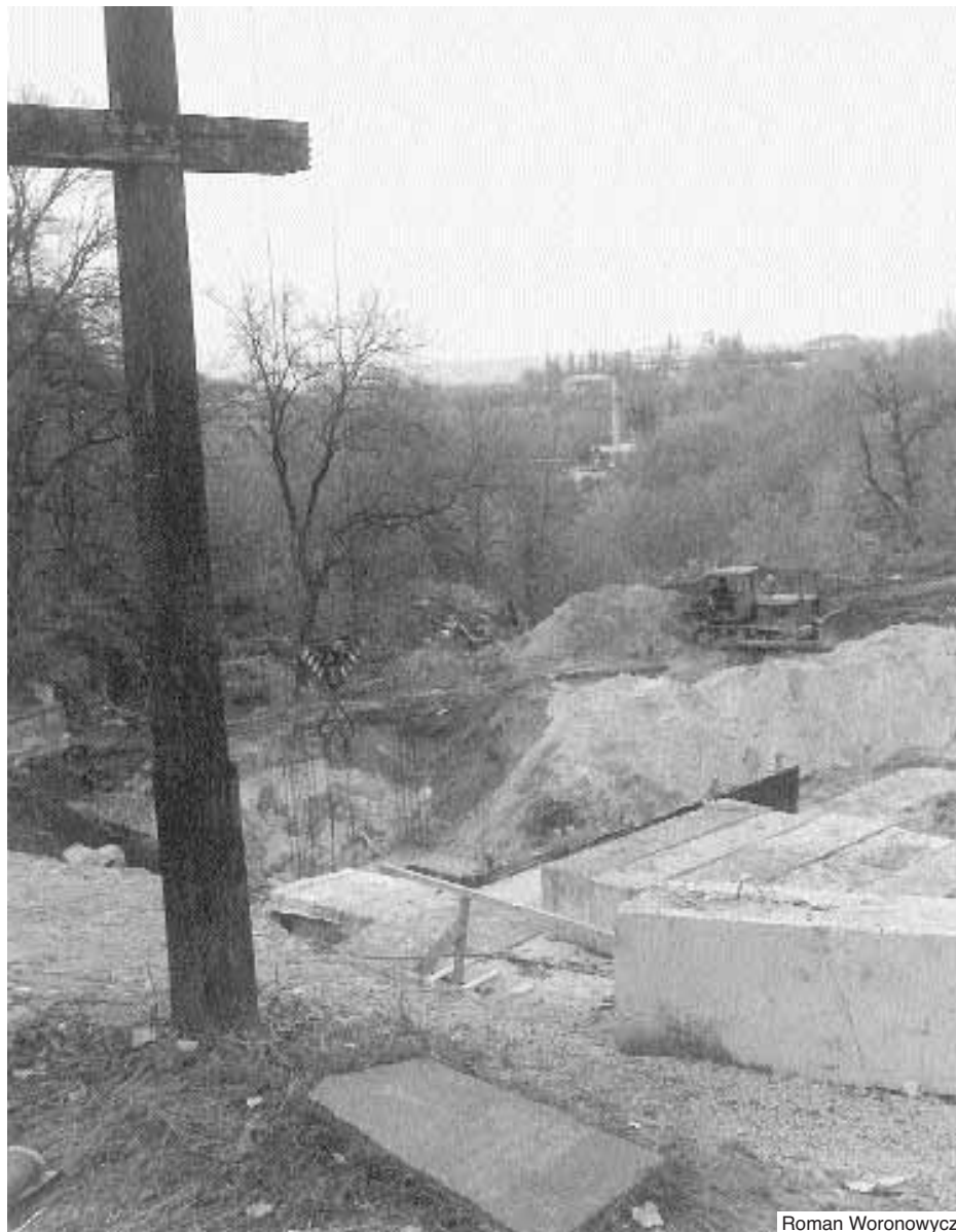
A view of the construction site located on a Kyiv hilltop.
