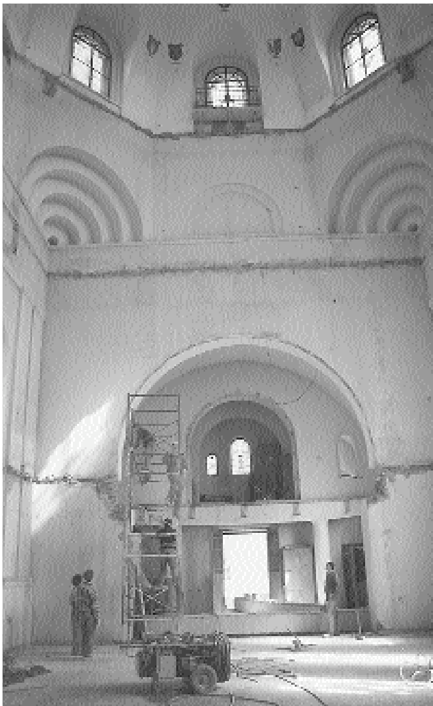
A view of the church's interior as it undergoes restoration.
