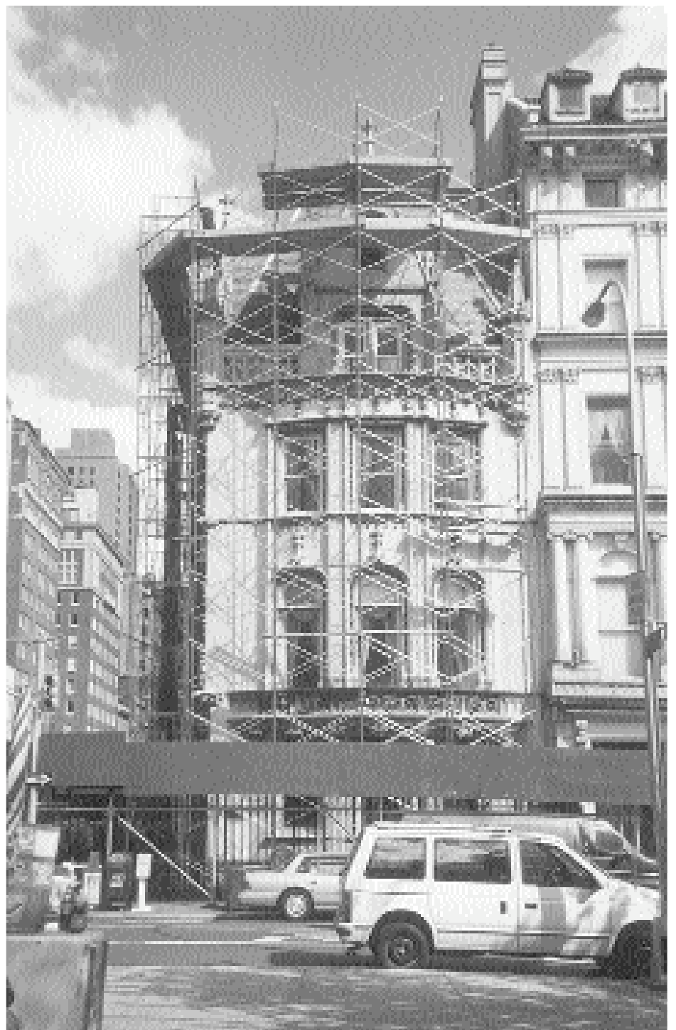
The Ukrainian Institute of America in scaffolding as it undergoes renovation.
