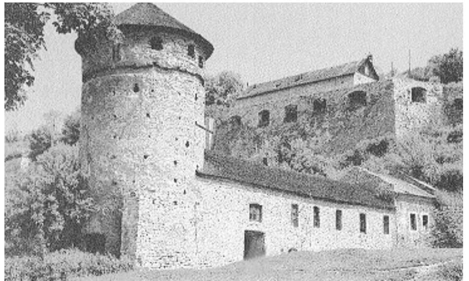
The Ukrainian Gate, located in the bottom of the gorge near the southern edge of Kamianets-Podilskyi, worked along with the Polish Gate to raise or lower the water level within the Smotrych River gorge during times of siege. Limited excavations were conducted at this spot in 1994.
