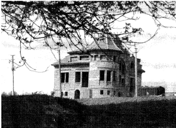
A new house under construction near Chernivtsi.
