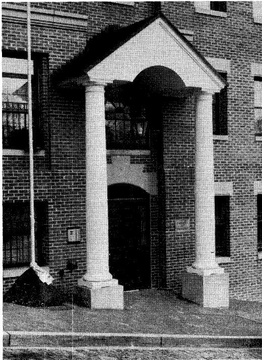
The portico and main entrance to the historic building.
