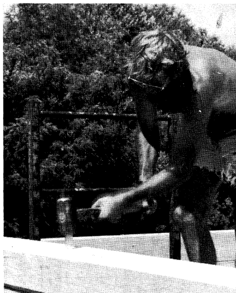
A wooden peg is driven into a log.
