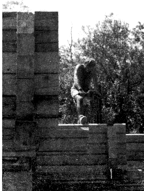
A craftsman prepares the hemlock logs for a wooden peg.
