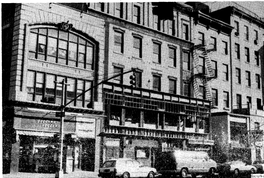
A look down Second Avenue between St. Mark's Place and Ninth Street shows work in progress at Ukrainian National Home.
