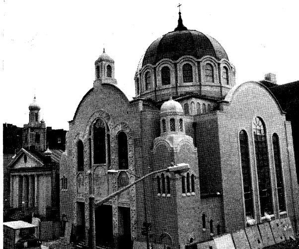
The new St. George's, right, dwarfs the older structure, left.
