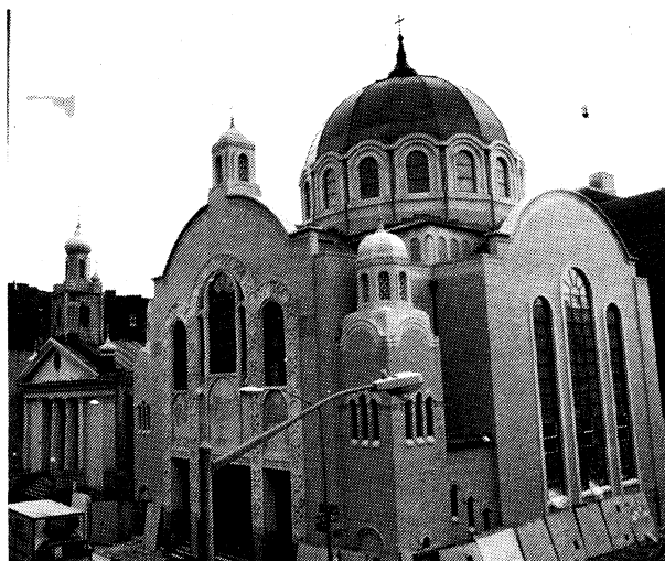
The new St. George's, right, dwarfs the older structure, left.
