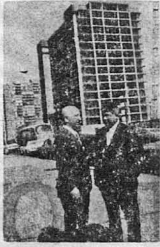
Michael Yarosh (right) chats with UNA President Joseph Lesawyer as they inspect construction sites of the UNA skyscraper and the Paulus Hook Towers in Jersey City.
