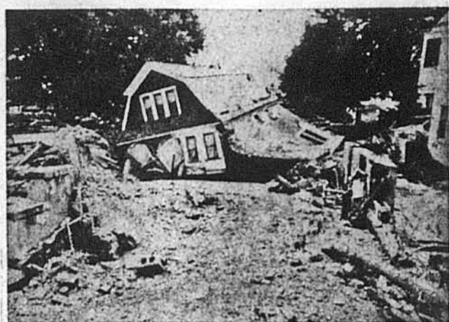
Photo above shows one of thousands of houses across the Wyoming Valley in Pennsylvania, destroyed by the floods in the latter part of June. Among the thousands left homeless are hundreds of Ukrainian families, many of them members of the Ukrainian National Association. It was last Friday, that the Executive Committee of the UNA, after a fact-finding mission by President Joseph Lesawyer and Assistant to the Secretary Stepan Hawrysz, designated $10,000 for relief of UNA families and called for a fund drive to help UNA members in the area.
