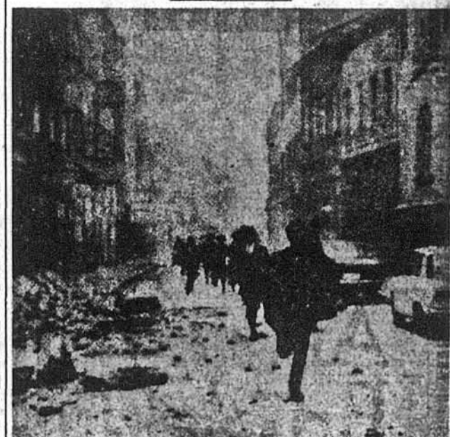
Banja Luka during earthquake.
